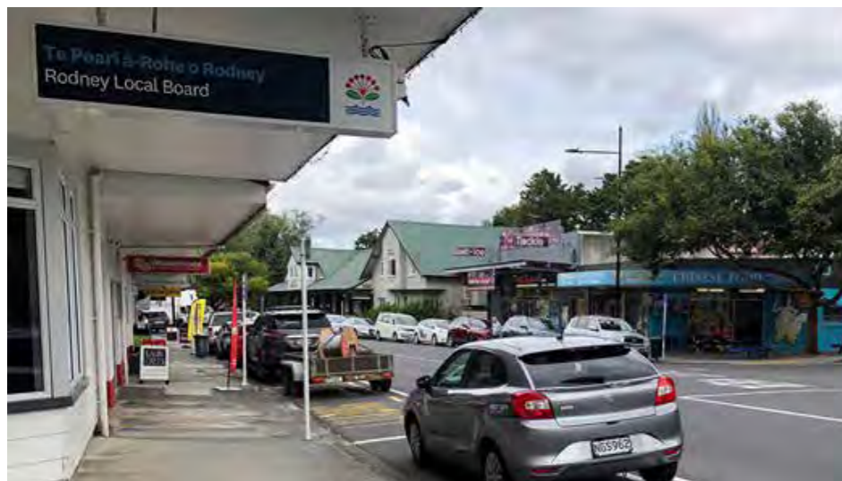
Photo Source: Our Auckland 3 March 2023 The new Rodney Local Board office.
